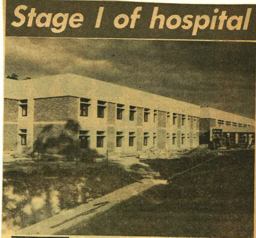
PICTURED is Stage I of the new Gosford District Hospital which is due to be completed late in 1979, and should be ready for occupation in February 1980. It is located on the southern side of the present hospital and is linked to it with an underground tunnel. Stage one consists of an operating theatre suite, accident and emergency department, four x 30-bed wards, temporary ICU/CCU, kitchen area, courier and communications area, admissions-discharge area, patient transfer area, and plant room.
